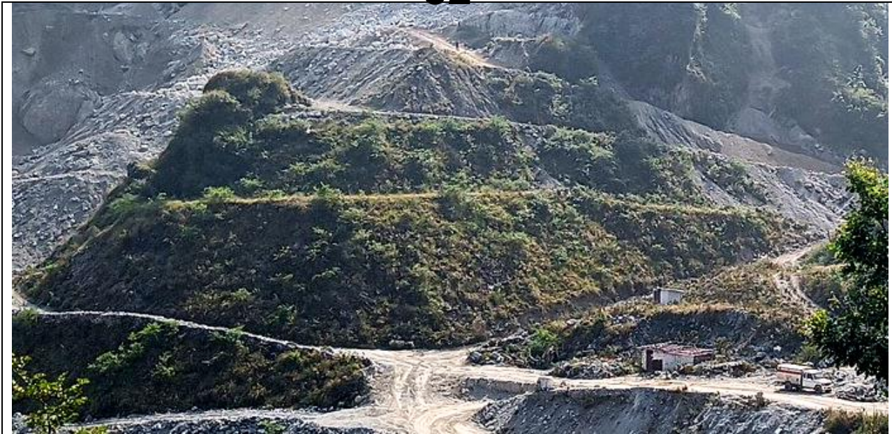
Photograph no. 7- Shows status of filled old dumping yard of M/s Bohar lime stone mine stabilized with plantation
